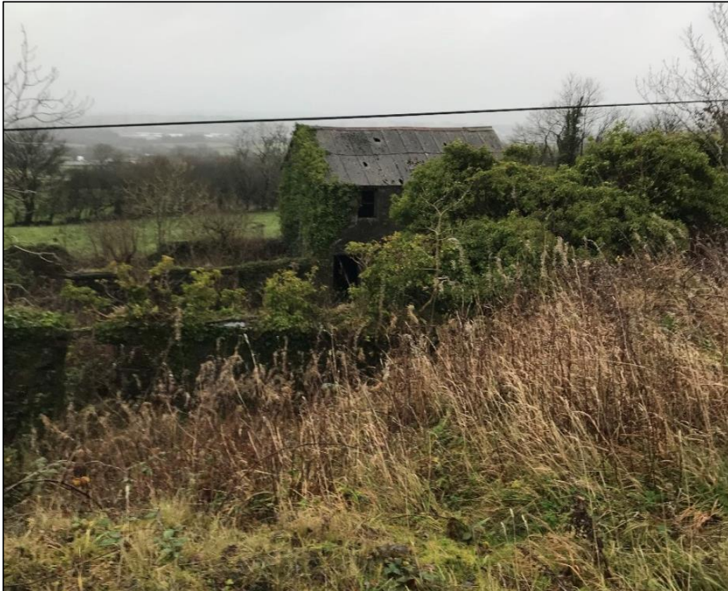
Figure 4.2 Abandoned building with asbestos containing materials in roof now used as a bat roost
