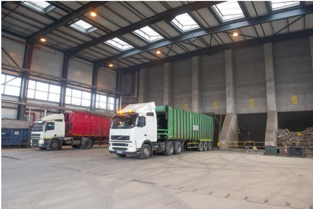
Fig 3.10 HGV reversing to waste bunker at Indaver's Co Meath EfW facility
