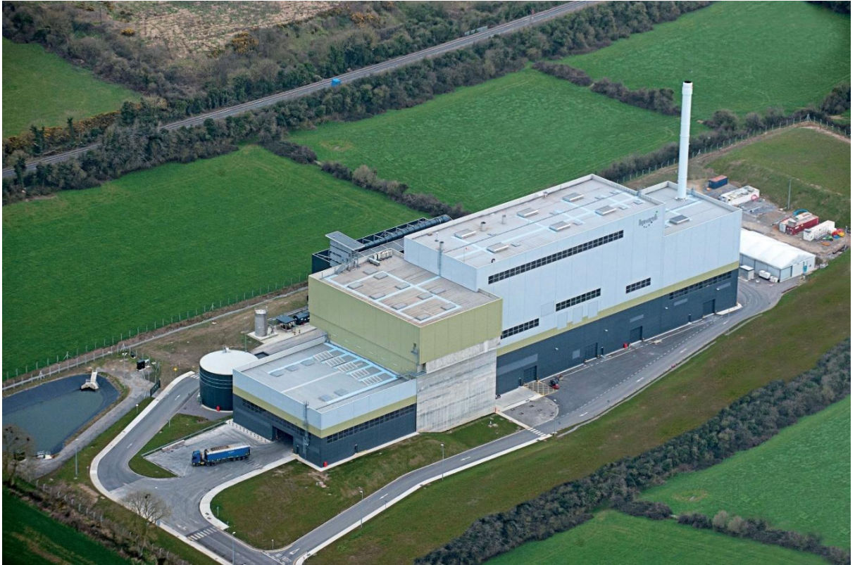
Fig 3.9 Indaver's Energy from Waste facility, Co. Meath
