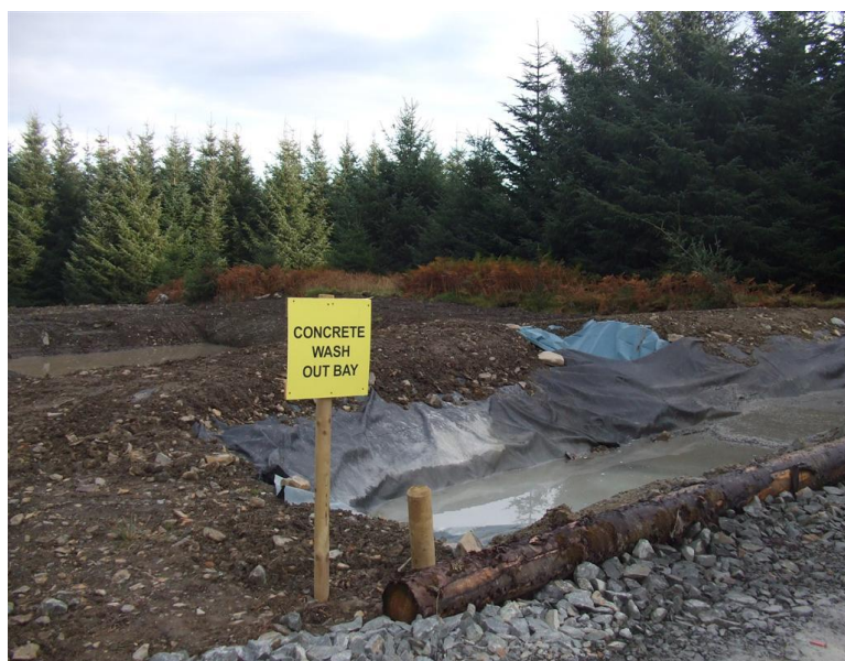
Figure 16 Example Concrete Washout Pit
