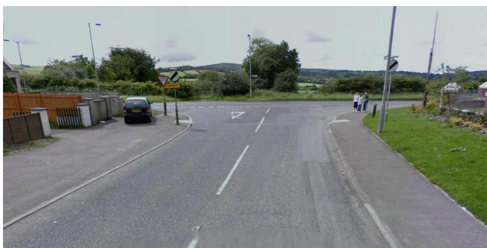
Figure 14 – Hightown Road junction with Hydepark Road
