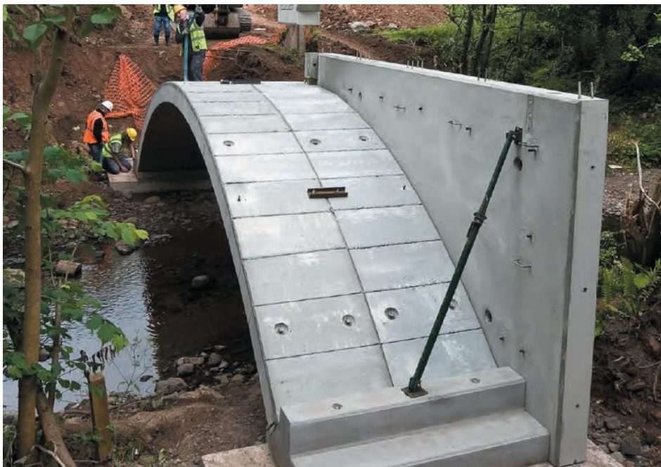
Figure 4 - Flexi-arch construction over a Waterway
