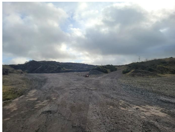
Figure 8.2 Storage of Road Planings
