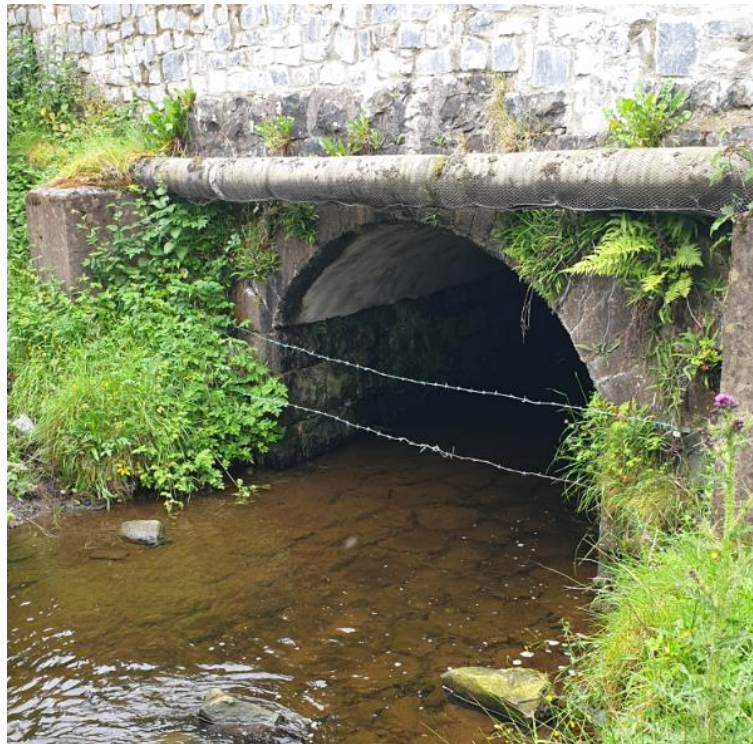
Figure 4.5: Southern Face of the Existing Flush Bridge
